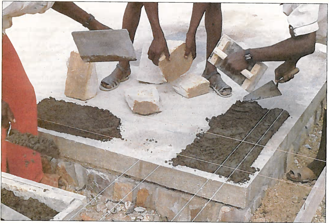
Tim Olson taught local workers how to build straight walls
