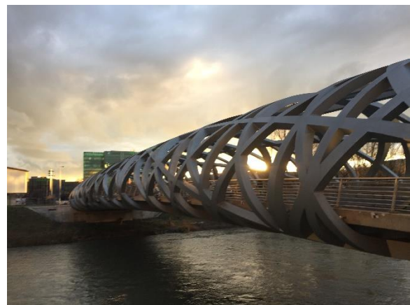
Fig 6. Hanswilsdorf Bridge in Geneva
