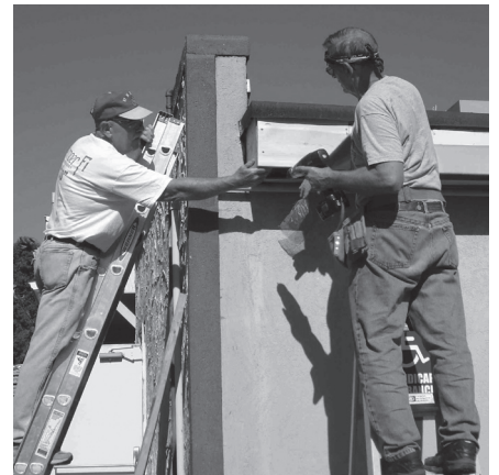
The 2007 Day of Caring resulted in some much-needed repairs
