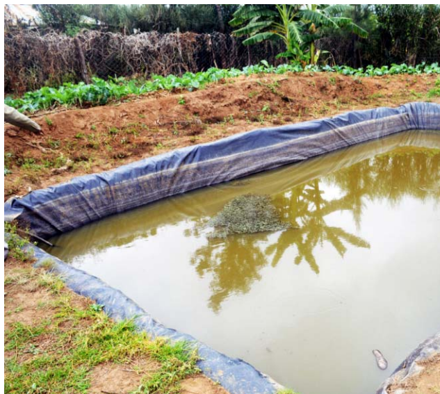
Dam liners enable small-scale farmers to collect rainwater for irrigation during dry seasons. Photo: D.Solie
